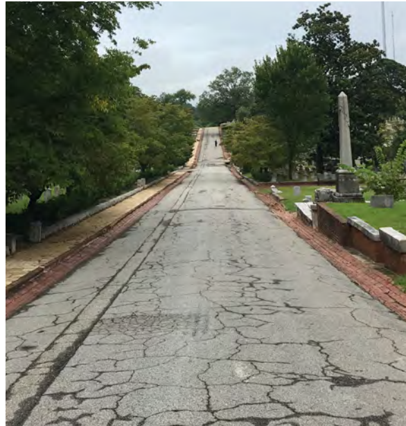
Updates to the watering system in the 1990s are evident in the patched asphalt of Old Hunter Street Drive.
