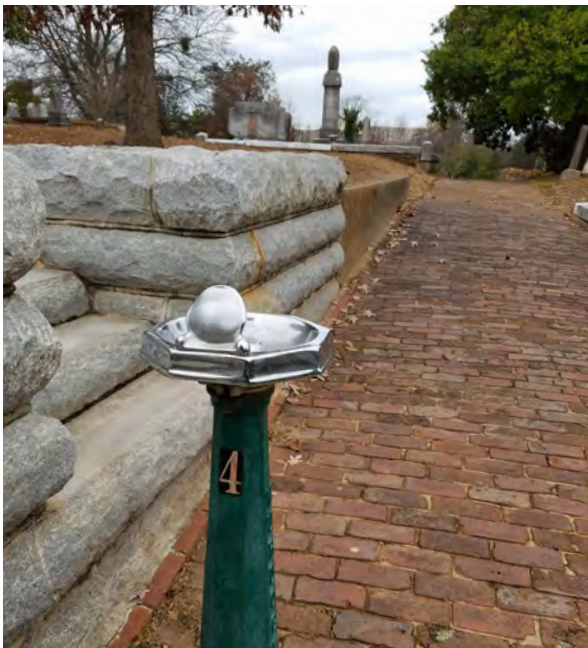
One of the nine sanitary drinking fountains installed in 2000.
