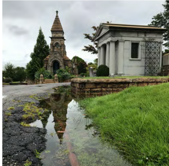
Standing water north of the Bell Tower. This area frequently sees heavy vehicular traffic and frequent roadside parking.
